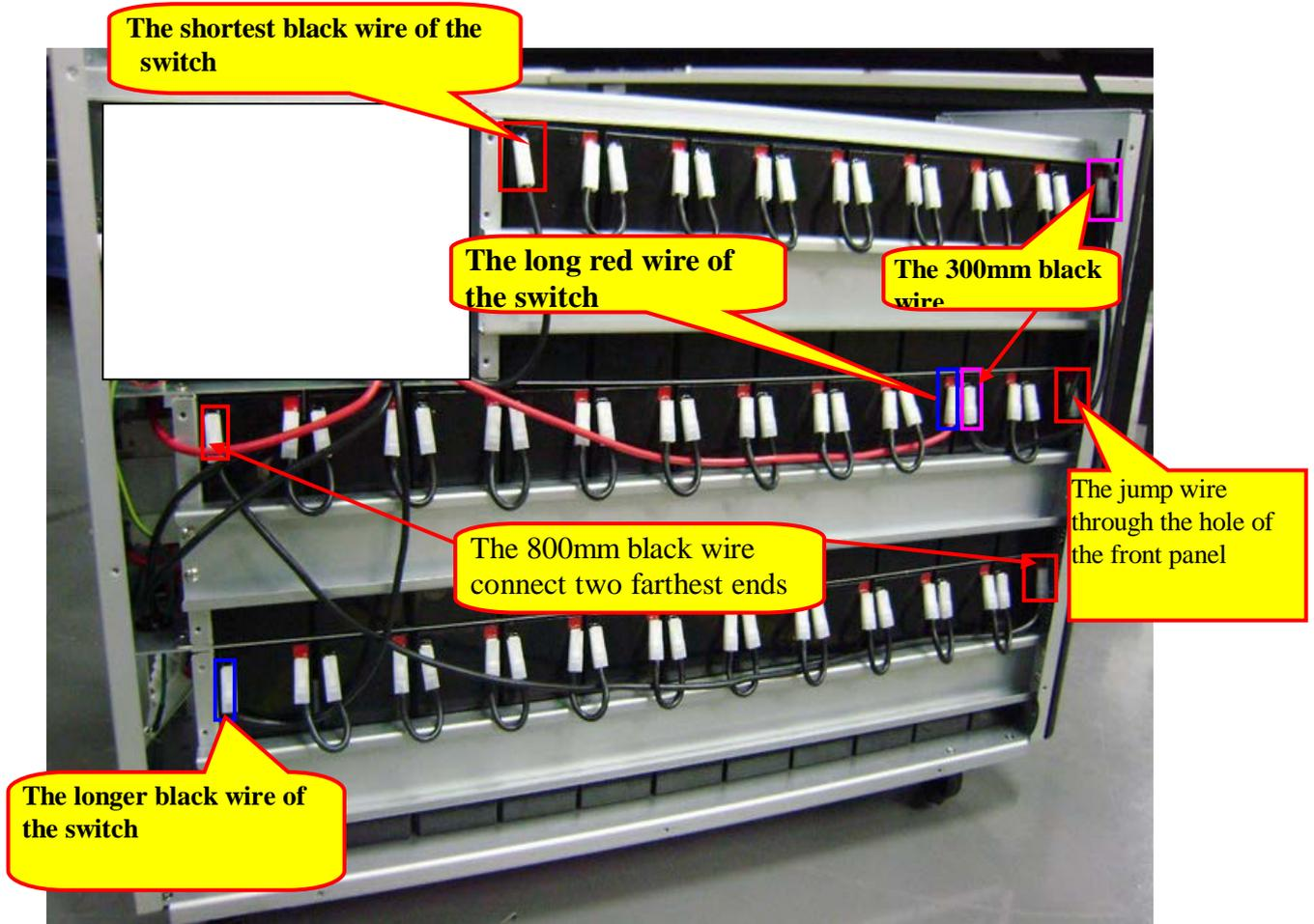
1. Insert the battery jump wires (as picture).
