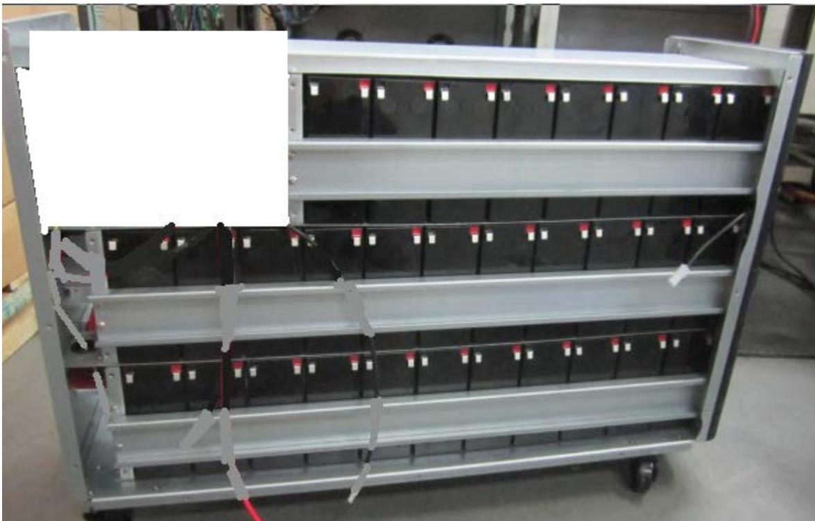
1. Insert the battery jump wire (as picture).
